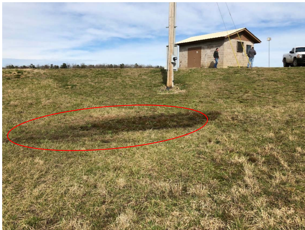
Figure 1: Excess moisture between Lagoon No. 1 and No. 2
