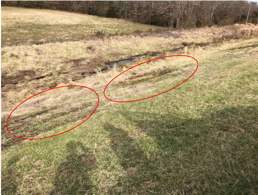
Figure 2: Excessive moisture on north slope of Lagoon No. 2
